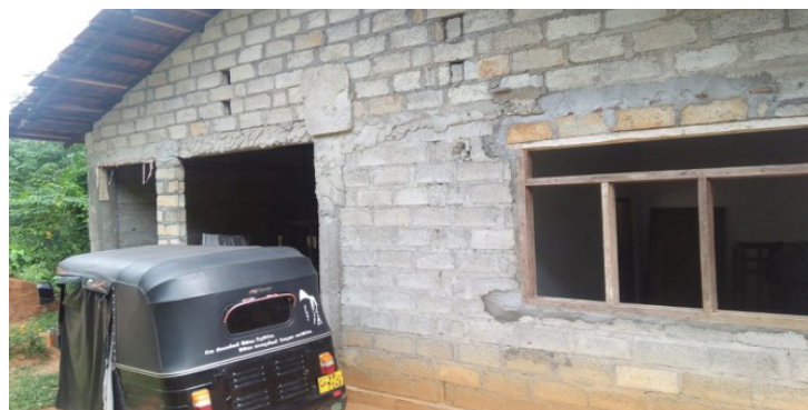
Photograph: Relocation housing in Construction, Sri Lanka
